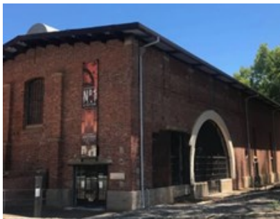
No 1 Pump Station
