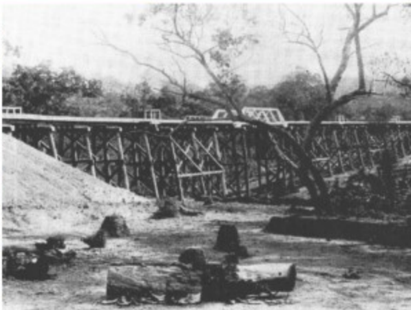
Jane Brook Railway Bridge c1896
